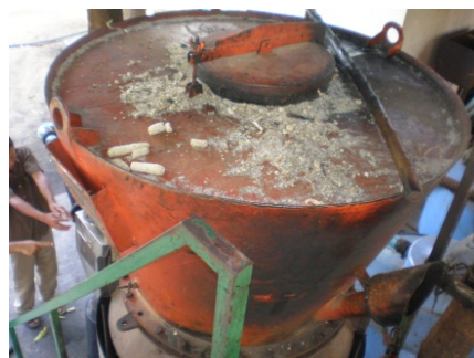
Fig. 3 Use of crop residues for electricity generation
