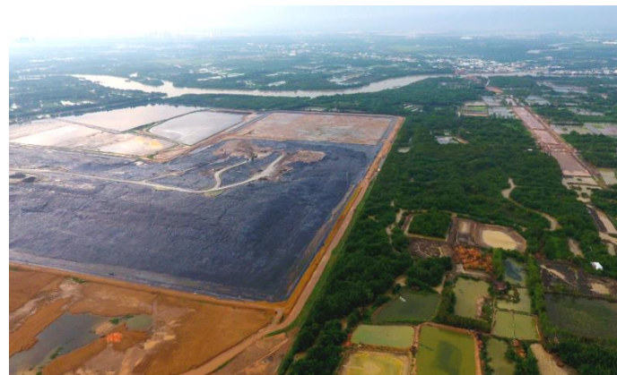
Da Phuoc landfill (Ho Chi Minh City) caused bad smelt to residential area
