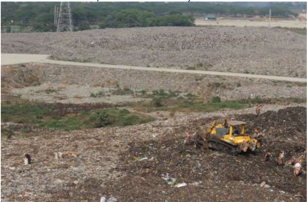
Matuail Sanitary Landfill Extension Area
