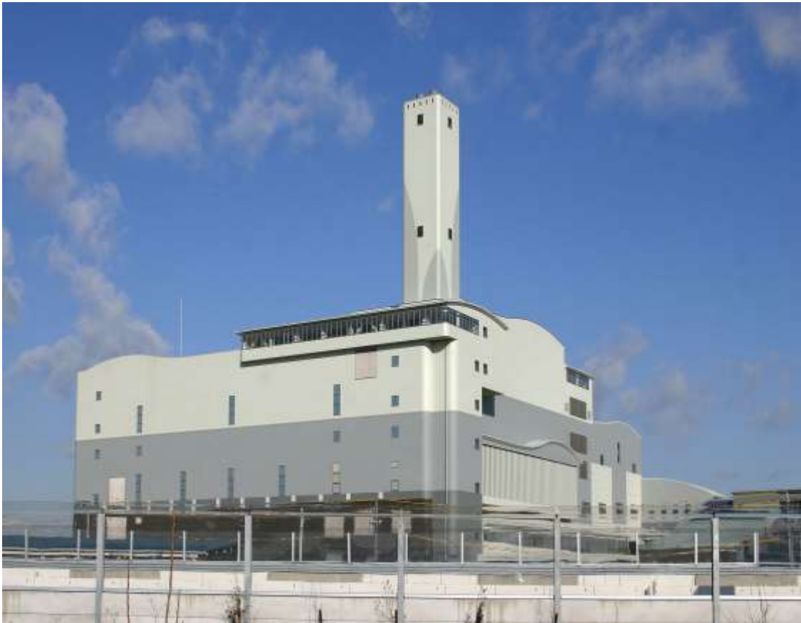
Togari Clean Center (waste incineration plant)
