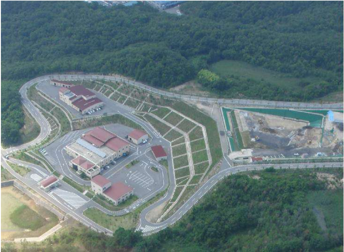
Green Clean Fujinooka (final disposal site)
