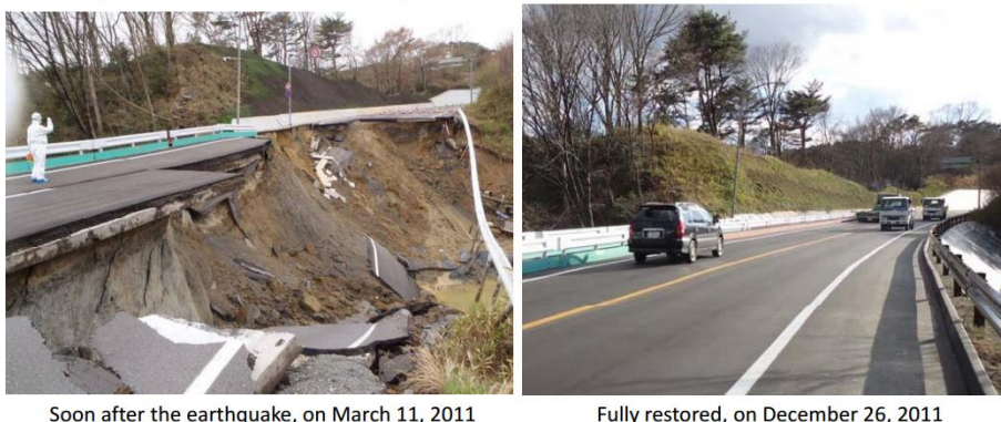
Figure 7: Damage to road embankments by the East Japan Earthquake (Sources: Motoda, 2013)
