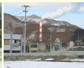
Taiheiyo Cement Ofunato factory
