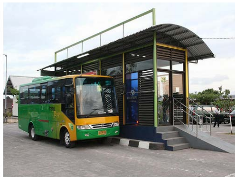
Figure 6. Integrated public parking area and bus shelter
